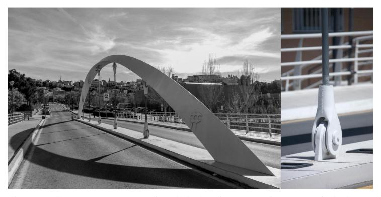
The structure of the project consists of a composite deck, a steel arch with a single span of 31.00 m between supports, five closed galfanized steel cables and load-supporting reinforced concrete abutments. The total width of the structure is 14.00 m, divided into a central part of 9.00 m for road traffic and two 2.50 m lateral parts for pedestrian use.
